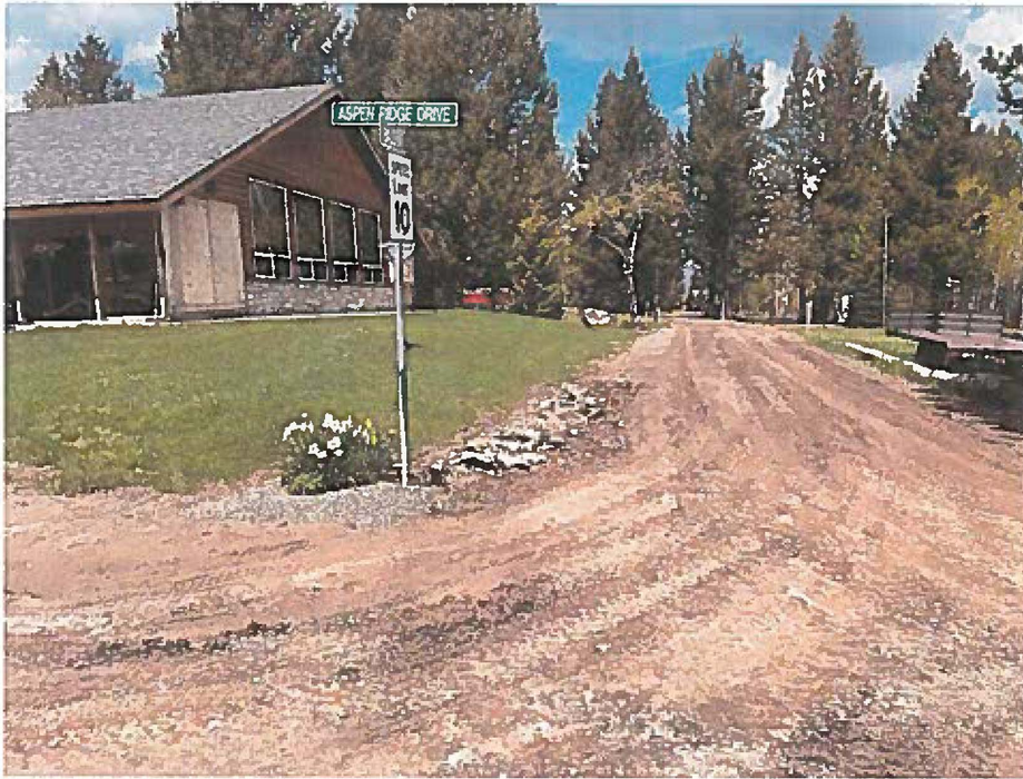
Photograph 1: Interstation of Balsam and Aspen Ridge where construction was occurring on May 18, 2023
